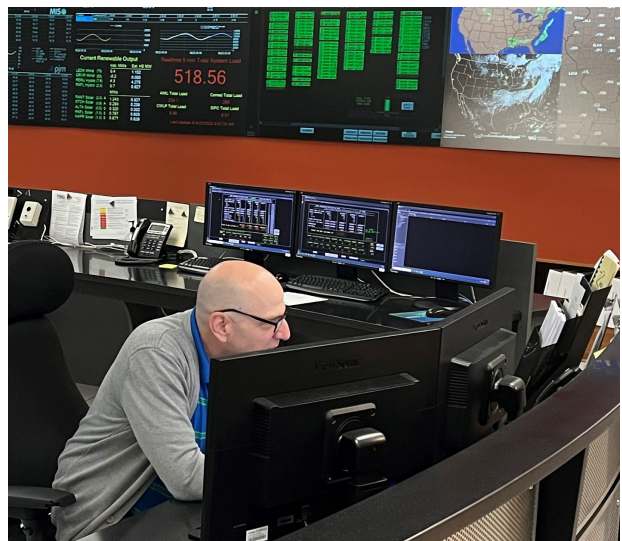
The IMEA state-of-the-art operations center is staffed 24-hours-a-day, 365-days-a-year to serve the needs of member municipalities.
